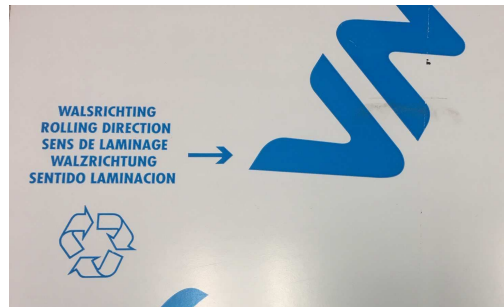
The Rolling Direction arrow indicated on the VMZINC Protective Film
