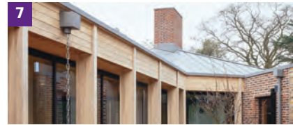
John Morden Centre – Day Care Centre
