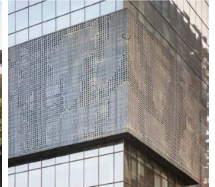
Project : Commercial Building, Noida System : VMZINC Perforation Panel Finish : QUARTZ-ZINC
