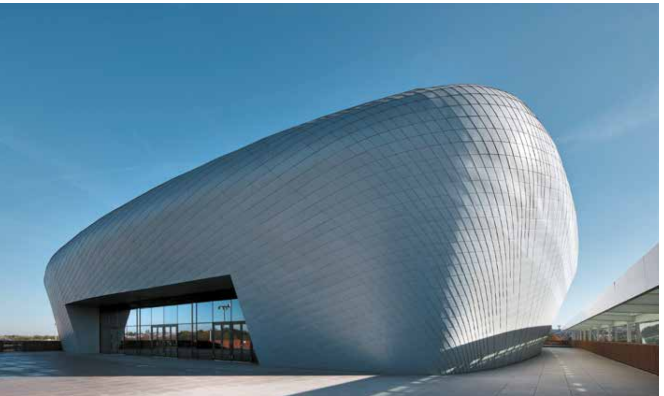
BREEAM • Docks Brussel • Architect : ART & BUILD • Brussels (Belgium)
